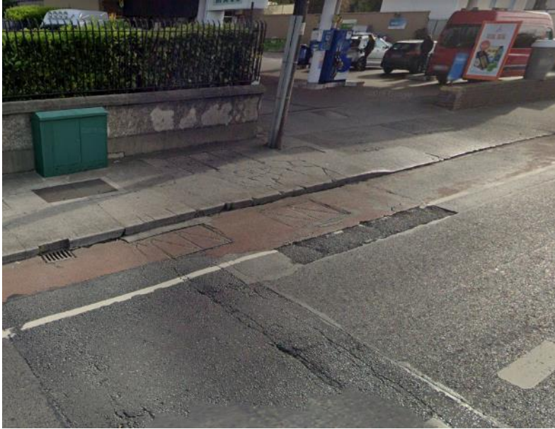
Figure 48: Surface Material - Navan Road
