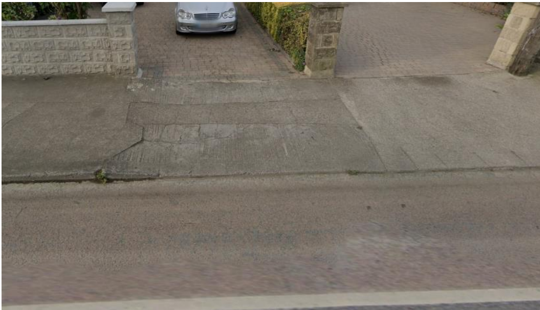
Figure 32: Poor Surface Material - Navan Road
