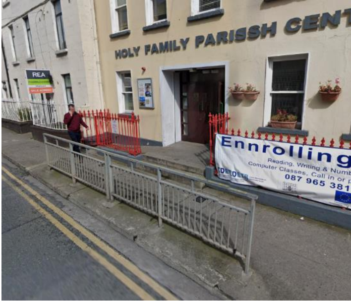
Figure 39: Guardrail - Prussia Street
