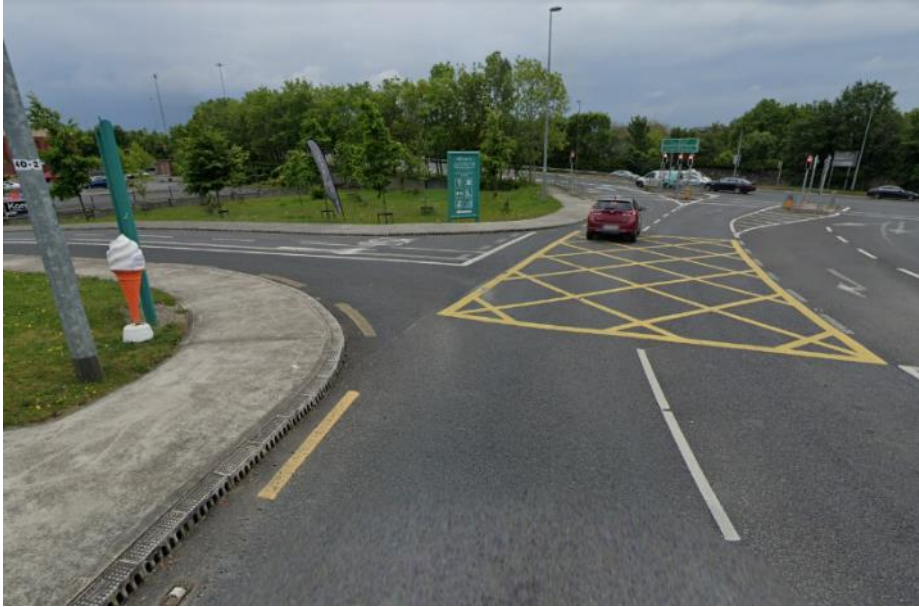
Figure 9: Pedestrian Crossing Point with no dropped kerb - Navan Slip Road
