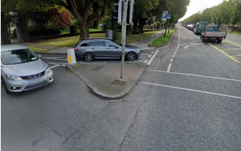
Figure 27: Limited or Missing Tactile Paving - Kempton Avenue
