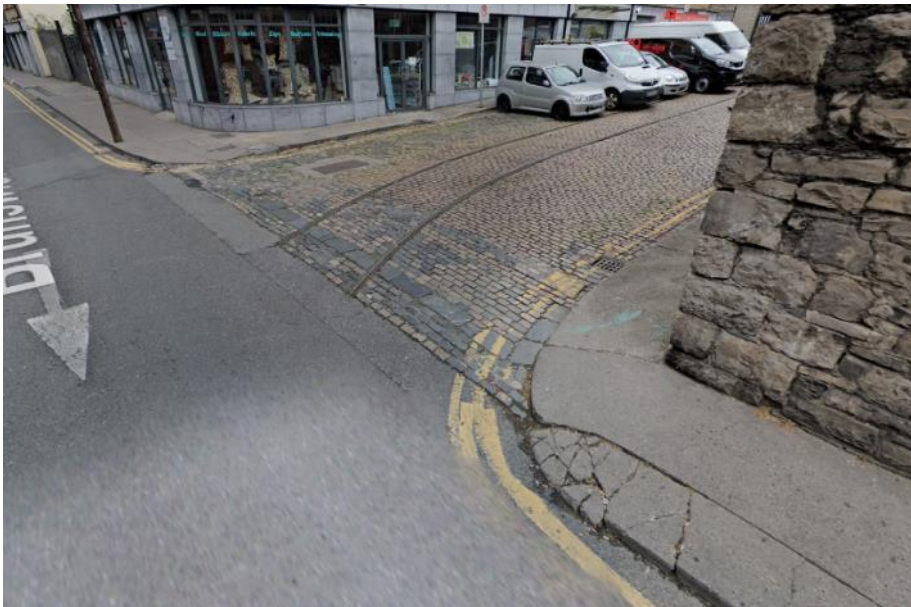
Figure 51: Surface Material - Brunswick Street North
