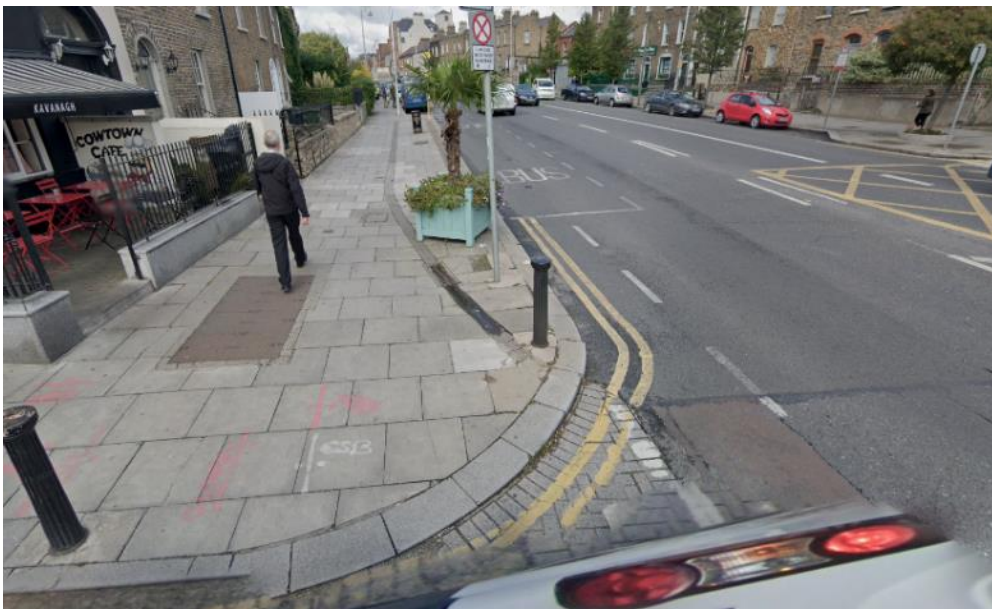
Figure 38: Footpath - Manor Street
