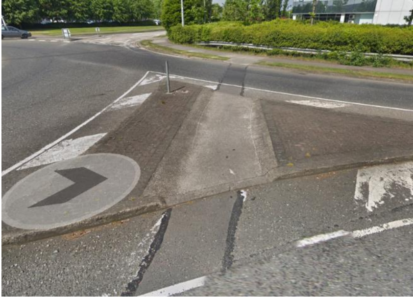
Figure 12: Tactile Paving - Missing tactile paving – L3020
