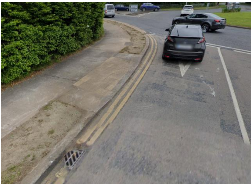
Figure 13: Insufficient tactile paving – Junction at Blanchardstown Shopping Centre
