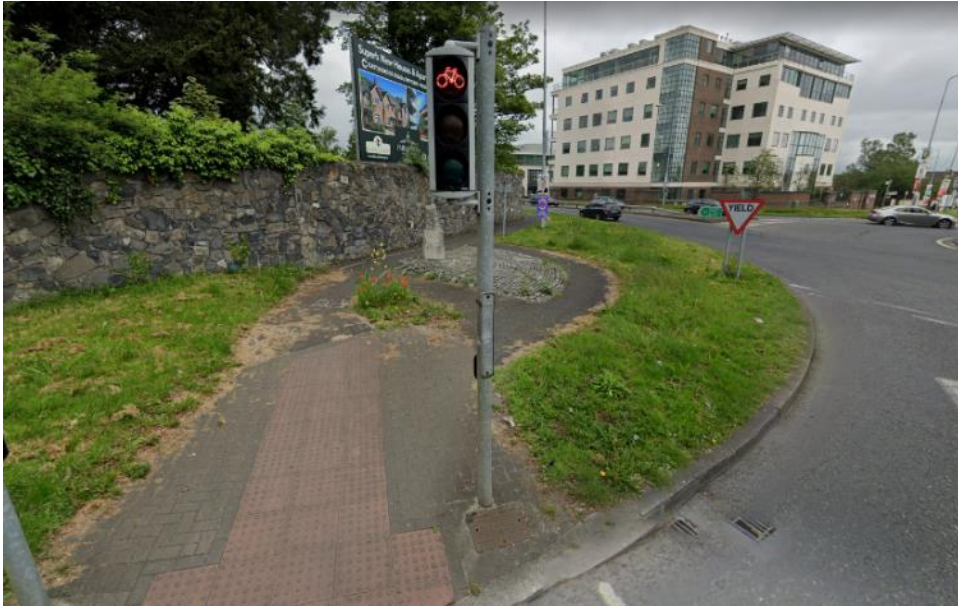
Figure 29: Shared Cycle track / footpath - Navan Road
