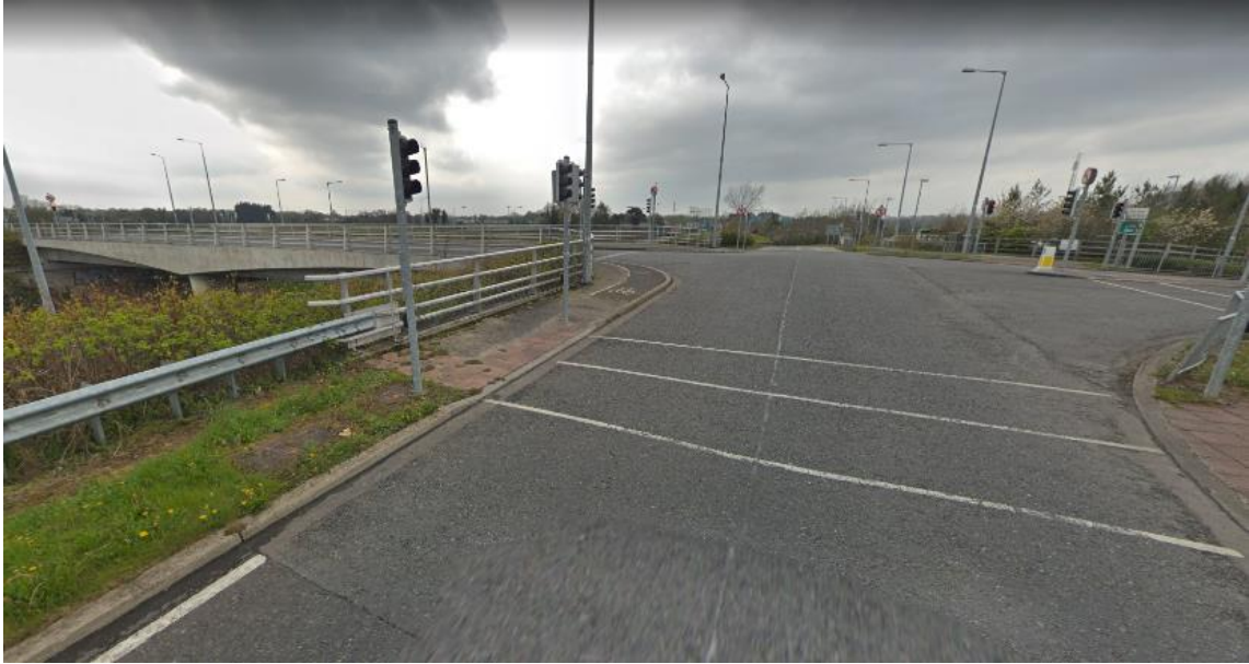
Figure 26: Controlled Crossing - Navan Road
