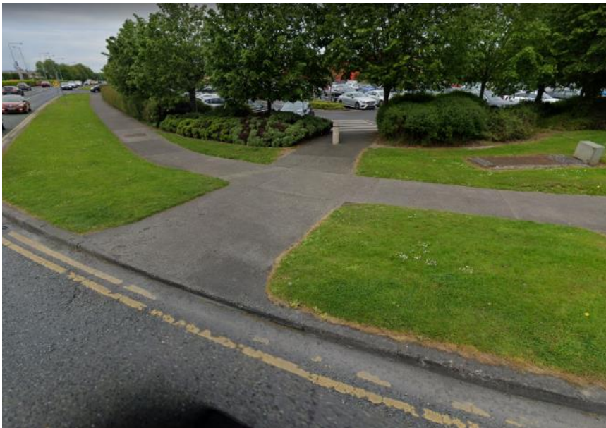
Figure 10: Pedestrian Crossing Point with no dropped kerb on curve of road.
