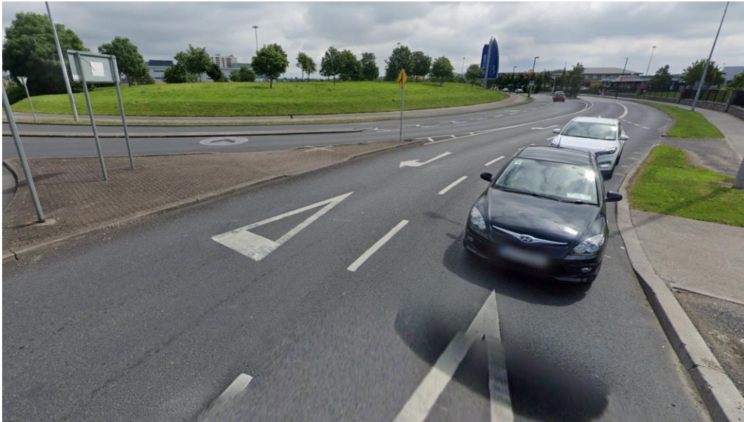
Figure 11: Pedestrian Crossing Point with poor layout – Blakestown Way Junction
