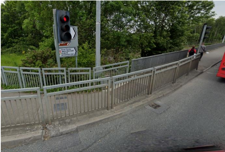
Figure 6: Guardrails - Snugborough Junction
