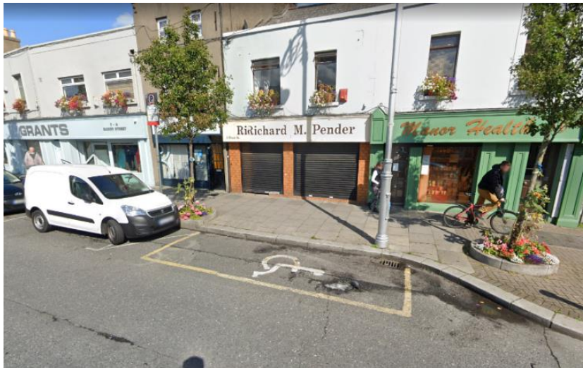
Figure 35: On-Street Disabled Parking - Manor Street
