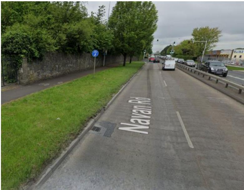
Figure 30: Shared Cycle Track / Footpath - Navan Road
