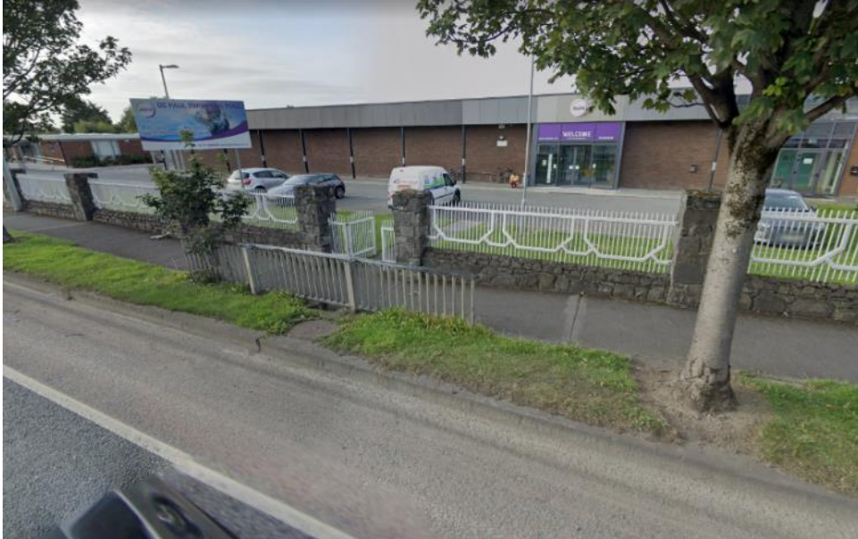
Figure 22: Guardrails - Navan Road
