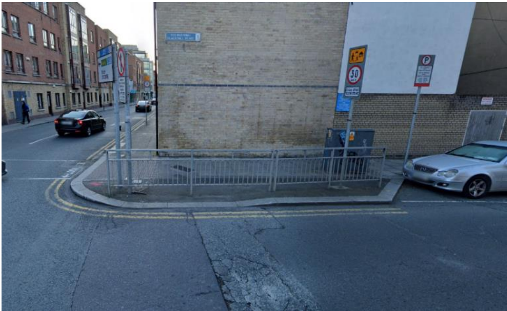
Figure 40: Guardrail - Blackhall Place
