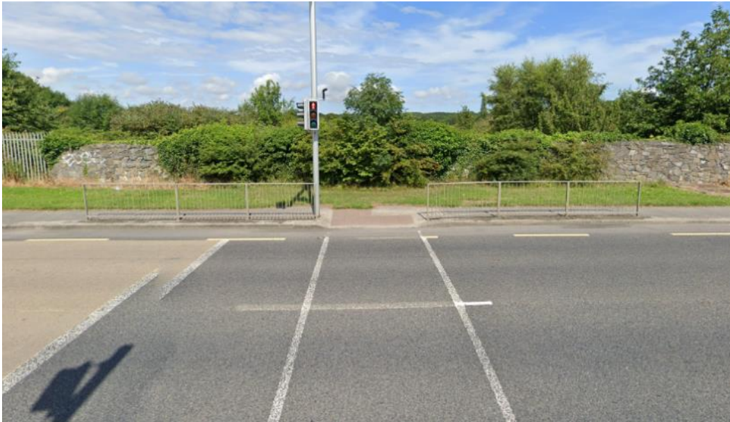
Figure 21: Guardrails - Navan Road
