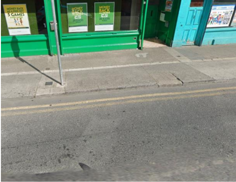
Figure 37: Footpath - Old Cabra Road
