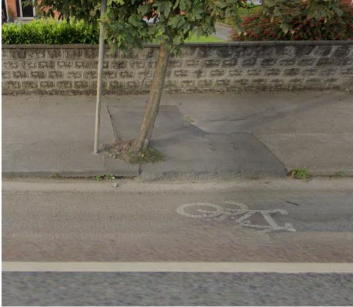
Figure 31: Poor Surface Material – Navan Road
