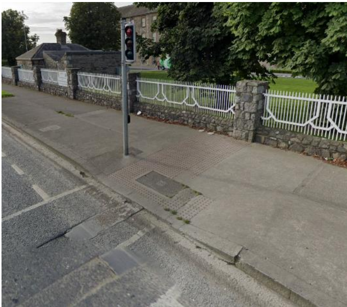
Figure 28: Limited or Missing Tactile Paving - Navan Road
